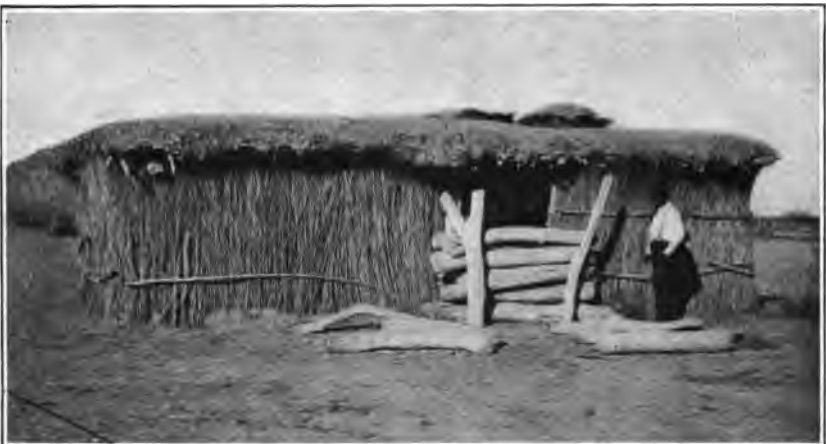
b WALLS OF RUSHES; COVERED WITH RUSHES AND ADOBE
